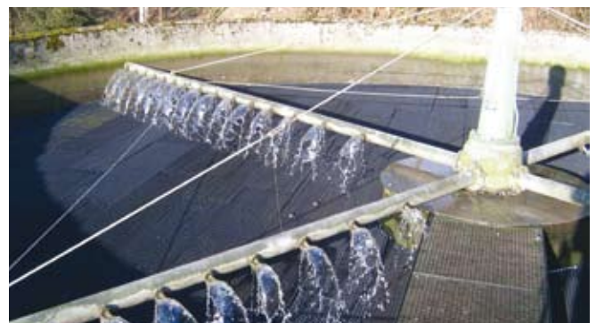
Upgraded Trickling Filter with gravity feed
