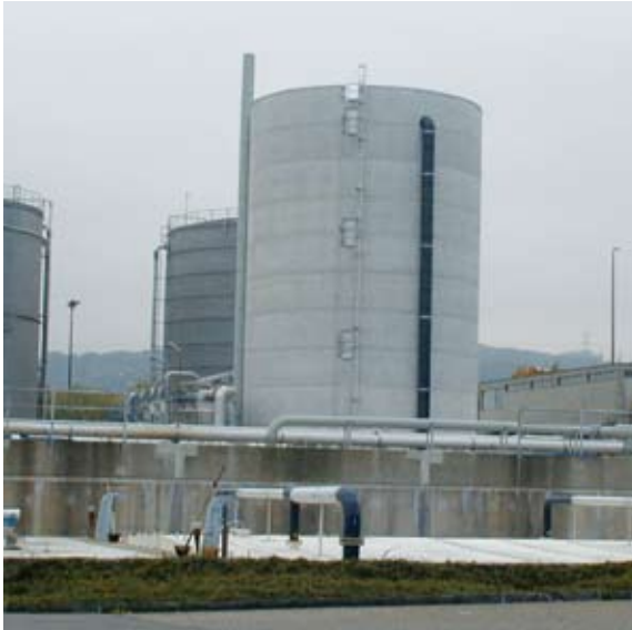
Trickling filter in industry with 16 m media depth Region Basel, Switzerland
