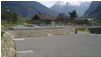
2H- GEOdek® Attinghausen, Switzerland: Road-runoff treatment
