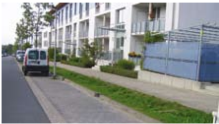
2H- GEOdek® Stormwater infiltration below a public parking area.
