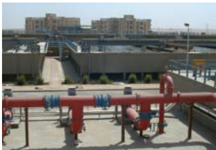
2H TUBEdek® Sheik Zayed City Plant: Potable water plant for satellite city of Cairo. Water source: River Nile. Treatment Capacity: 3 Mio Habitants.
