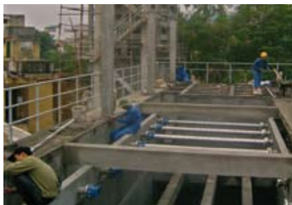
2H TUBEdek® Kim Lien potable water plant in the centre of Hanoi: Lamella clarifier equipped with TUBEdek®
