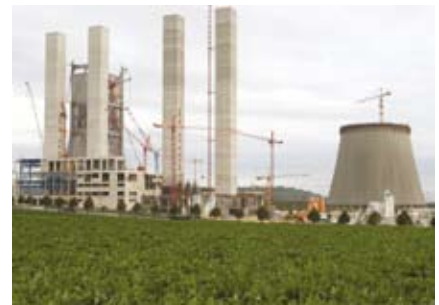
2H- PLASdek® Neurath, Germany: First installation of fills and drift eliminators (2008)
